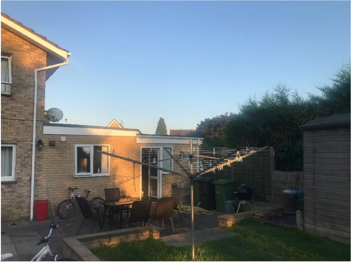
(1) View from No 23's rear garden looking to the Proposal's site (the East Garden)
